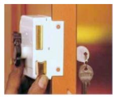
Installation Position of Rim Lock on Door
